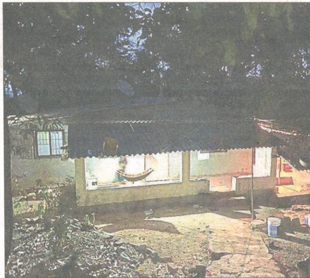
■ Jhamjad Pada, located in a remote hilly area of Gorai, got power more than a decade after they had first applied for a connection in 2008. The hamlet has been in existence for around 70 years. HT
