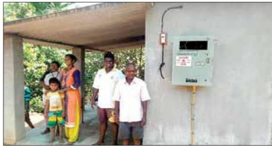
A tribal family poses alongside its newly installed electricity board
